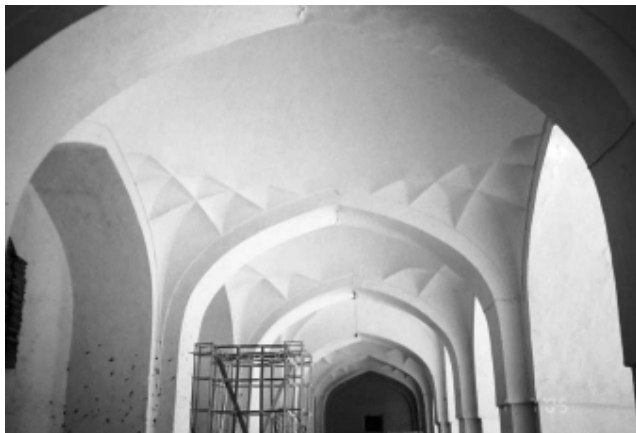
Plate-XIII: A View of Phase of transition of Cloisters with Ceiling, Akbari mosque
